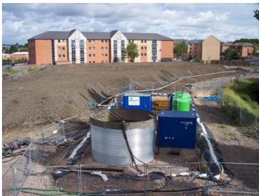
Bio-Pile and Water Treatment Plant
