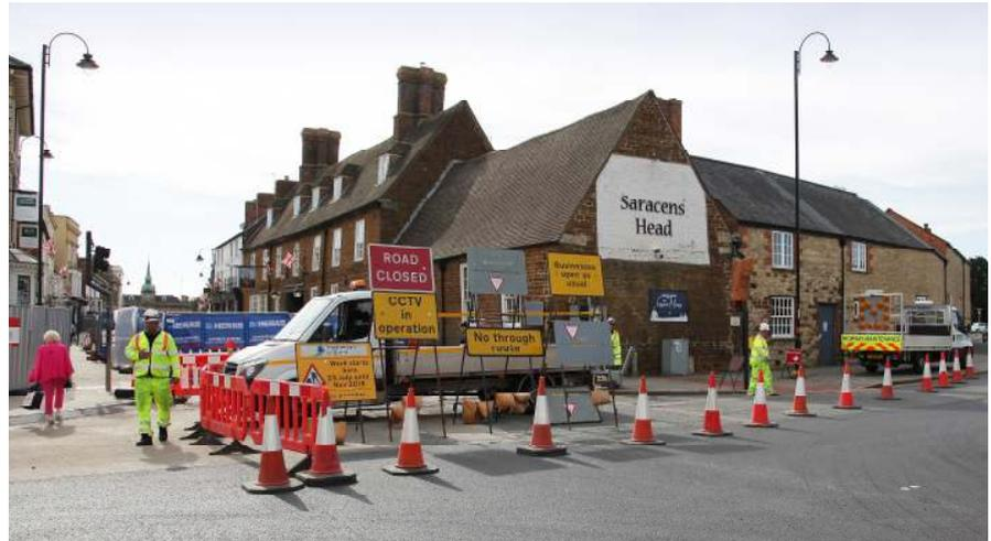
This was a high profile scheme involving essential maintenance work to 1.3km of the A5 Watling Street in Towcester, Northants to address various issues including poor highway drainage, extensive surface water ponding that was causing splash damage to properties and posing a significant risk to pedestrians, cracking and rutting of poor quality reinstatement to a 430 m long gas main trench installed in 2009 together with replacement of kerbs and footpaths damaged by vehicle encroachment.
