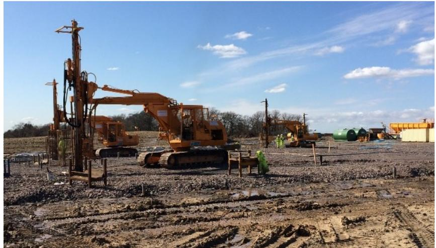
Contract to undertake shallow mine workings consolidation along the route of the M8 improvements being constructed by the Ferrovial Lagan JV in a DBFO contract for Transport Scotland.
